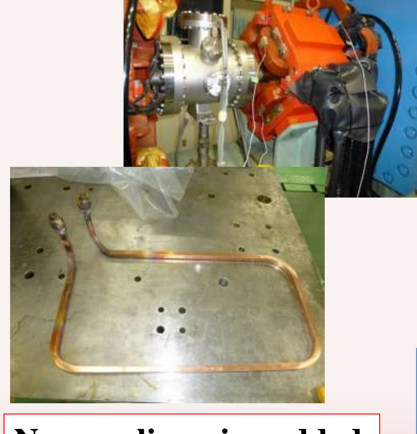
New cooling pipe added.
