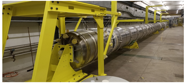
Figure 6: The lower beamline of the pilot sector after final alignment.
