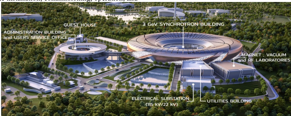
Figure 1: Overview of the Siam Photon Source II facility.
