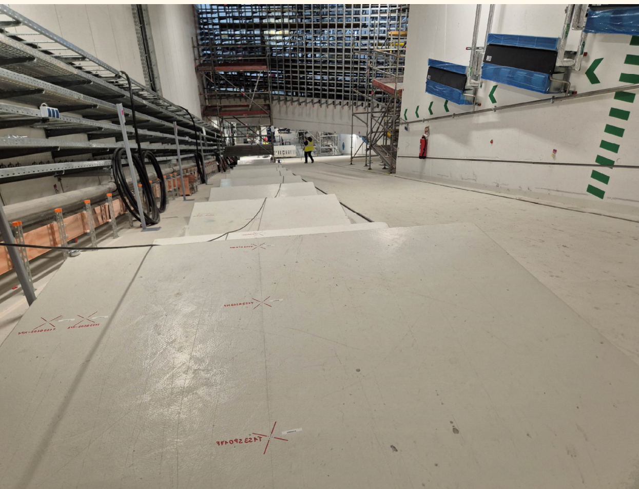
Highly challenging blue-lining on the 15° ramp leading to SIS100.
