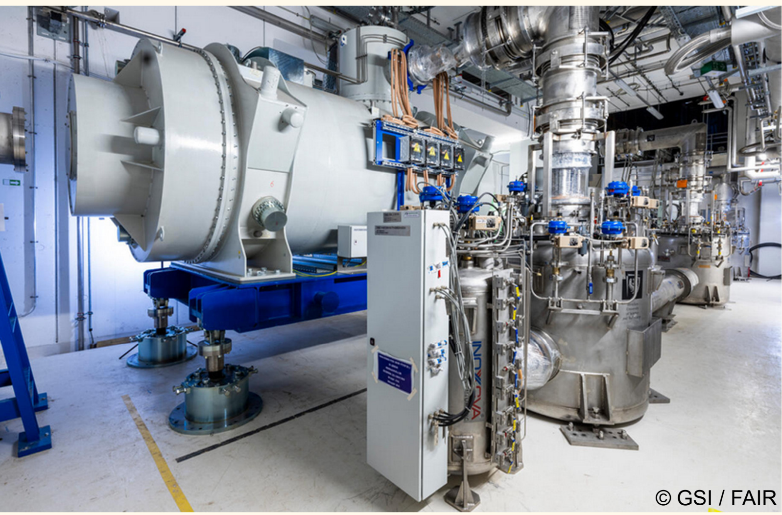
A multiplet in the Super-FRS pre-target area
