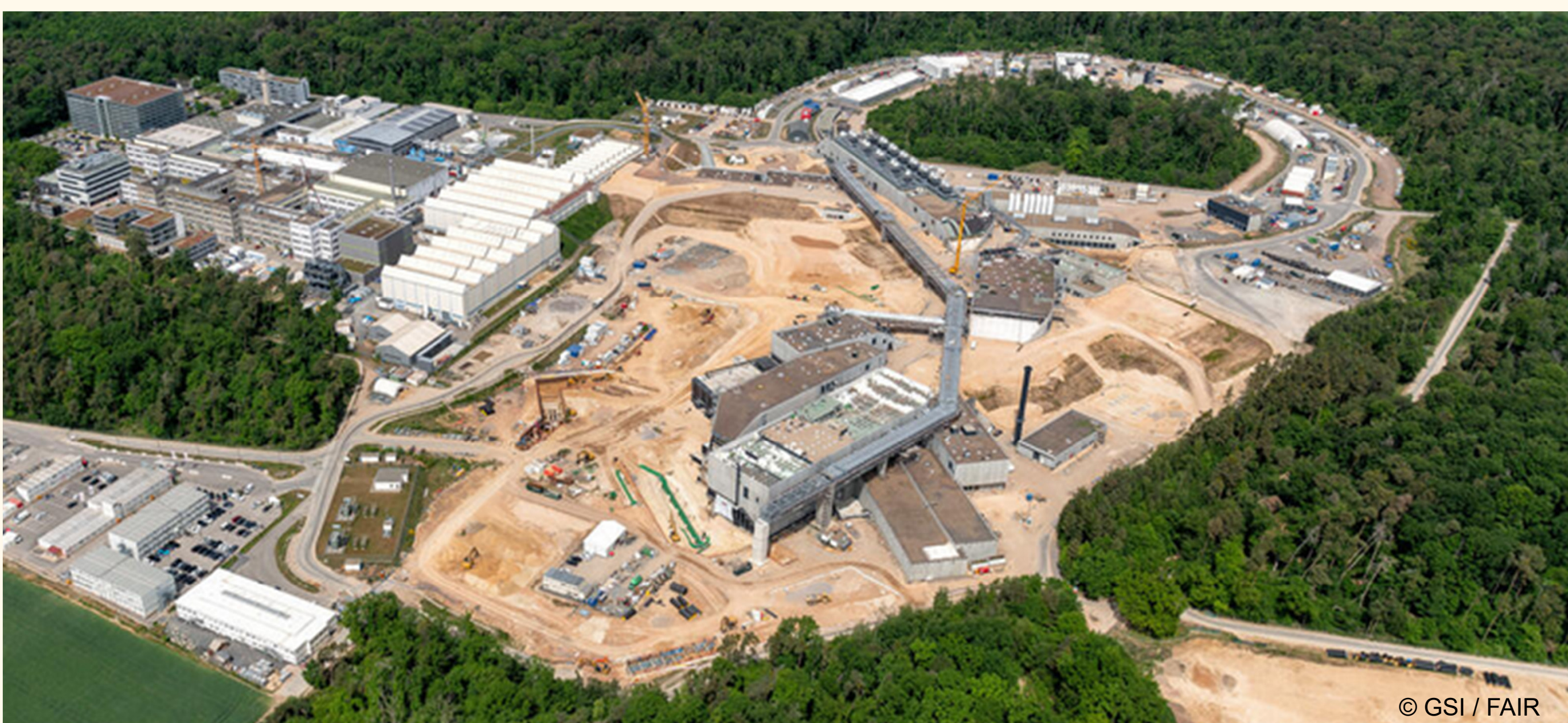
FAIR construction site – Overview 2026
