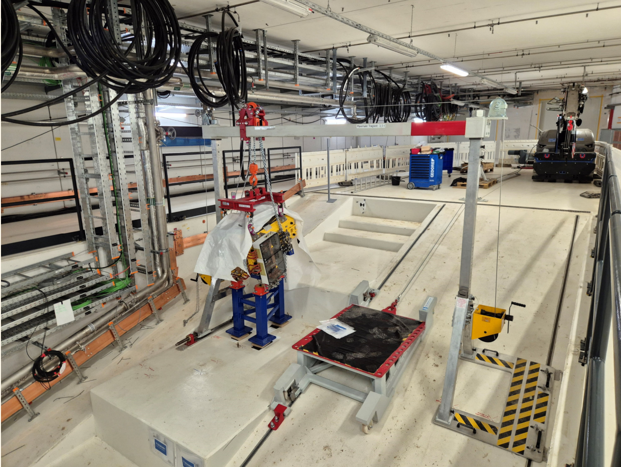
The first installation test of a normal conducting quadrupole on the 15° HEBT-ramp
