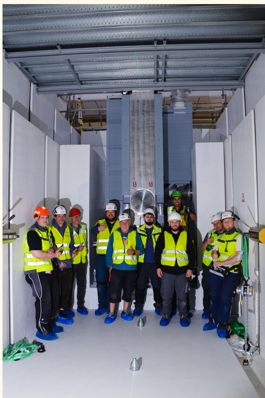
Super-FRS – Target Chamber installed
