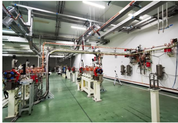
Waveguide system
