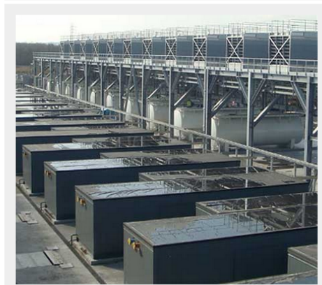
The Google data center in Belgium, which features no chillers and routes traffic to other facilities during hot spells. (Photo from Google)
