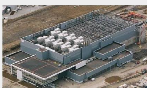
An aerial view of Microsoft's huge Dublin data center.
